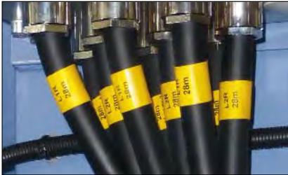
The printable, thin wall **TF21 heat shrinkable tubing** is used for clear marking of cables and lines, for example to mark the phase position of power cables or PE markings.
