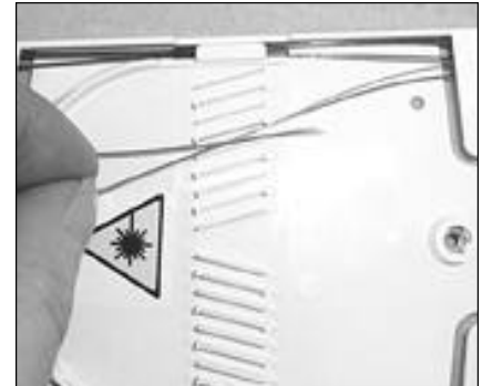
12. Splice the fibres using standard procedures
