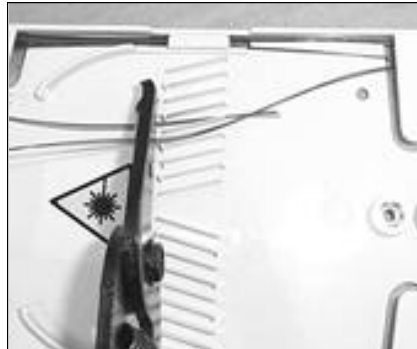
11. Cut the fibres on the opposite side of the fins.
