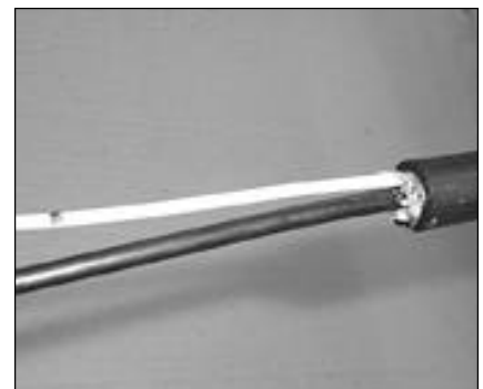
60. Mark each of the fibre units 70mm from the sheath butt position 'B'.
