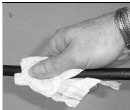
50. Clean the cable for distance of 4 metres.
