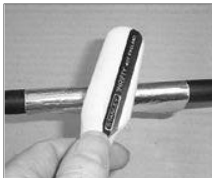
14. Rub the foil using a suitable tool.
