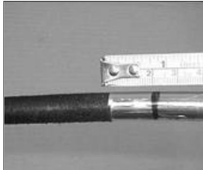
65. Mark the foil 20mm from position 'A'.
