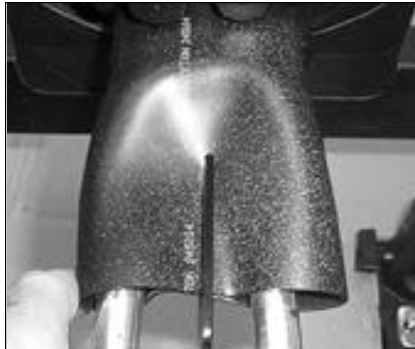
38. Separate the cables and insert the branch clip provided.
