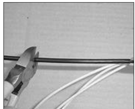
15. Cut the central strength member 150mm from position 'B'.
