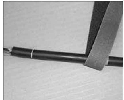
12. Abrade the cable between positions 'A' and 'D'.
