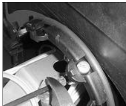
68. Cut the central strength member, 5 to 10mm from the anchor fixing.
