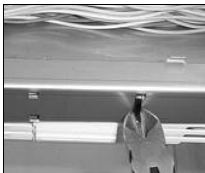
71. Cut the cable ties securing the fibre unit to the basket.
