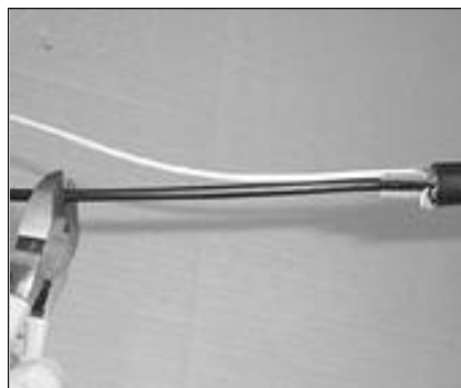
59. Cut the central strength member 150mm from position 'B'.
