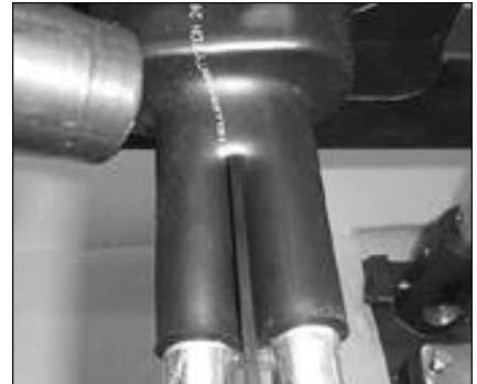
39. Recover the heatshrink on to the cable.
