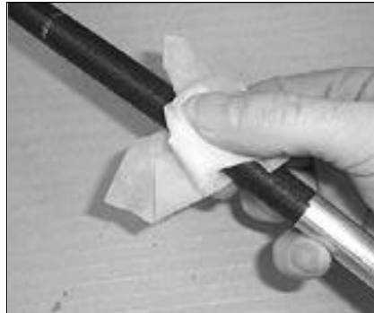
20. Clean the abraded area of the cable using an IPA wipe supplied.
